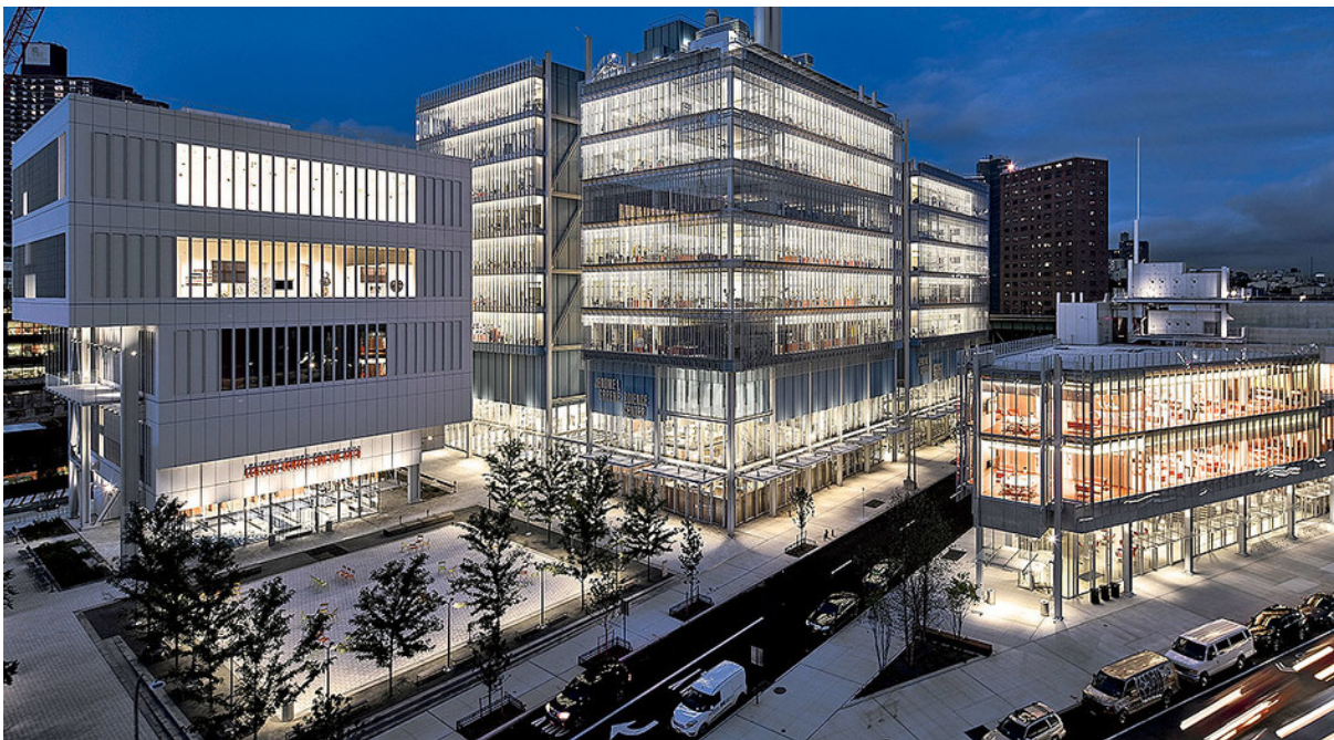
Manhattanville's first new facilities: the Lenfest Center for the Arts, the Jerome L. Greene Science Center, and the Forum. (Frank Oudeman)
