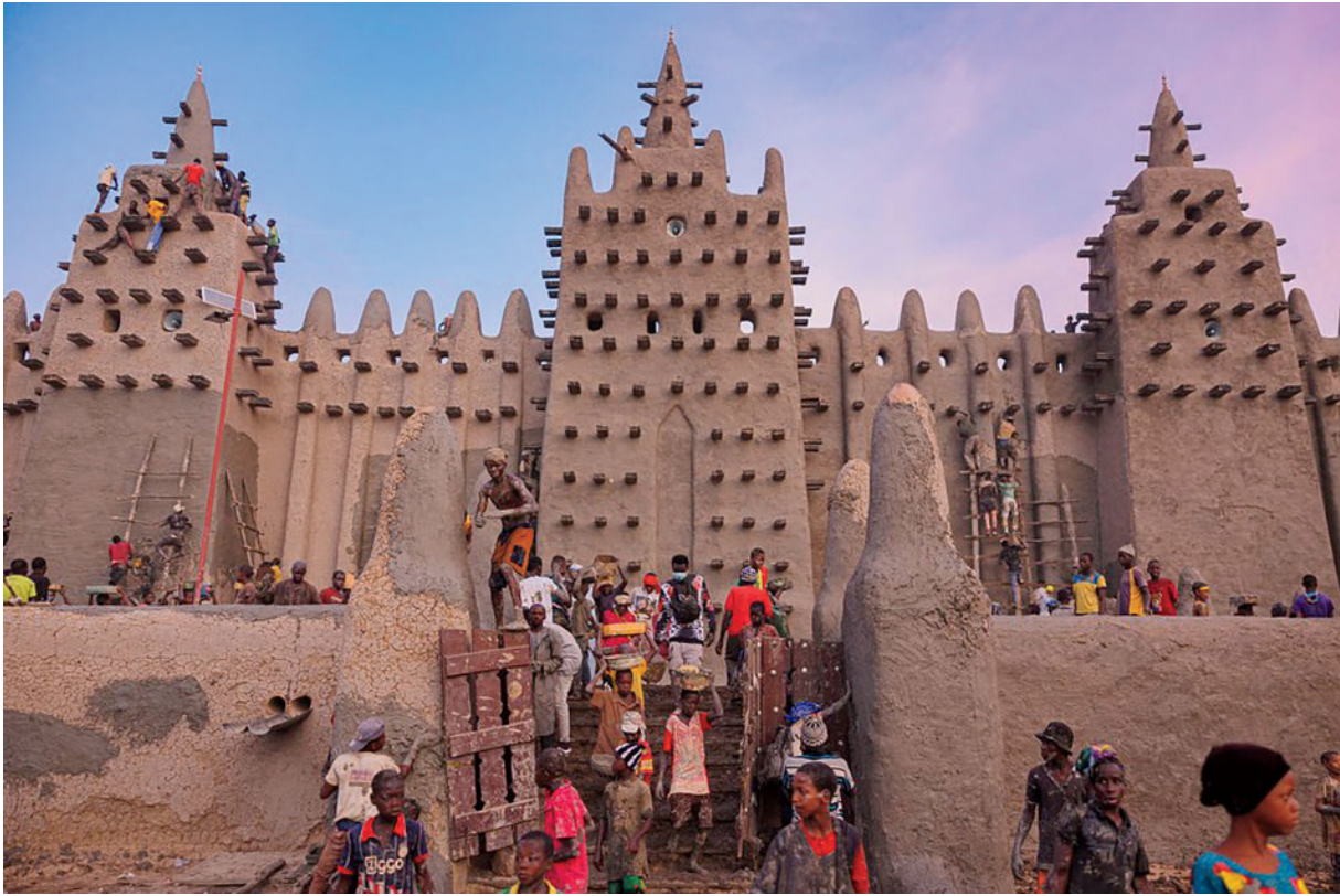
Replastering the Great Mosque of Djenné, in Mali. (Ousmane Makaveli / Getty)
