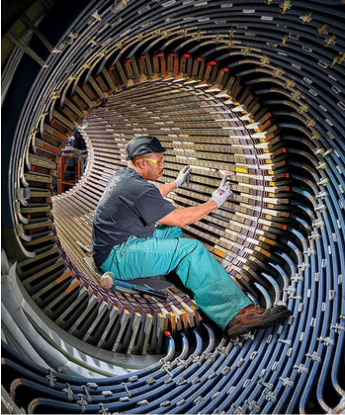
A hydrogen-cooled generator at GE Gas Power, Schenectady, New York.
