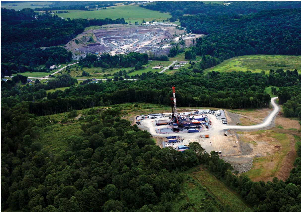
A natural-gas drilling site in northeastern Pennsylvania (Mark Ovaska / Redux)
