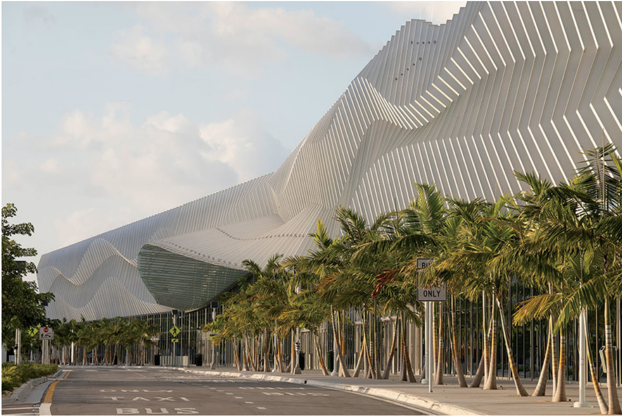
Robin Hill / Courtesy of Arquitectonica
