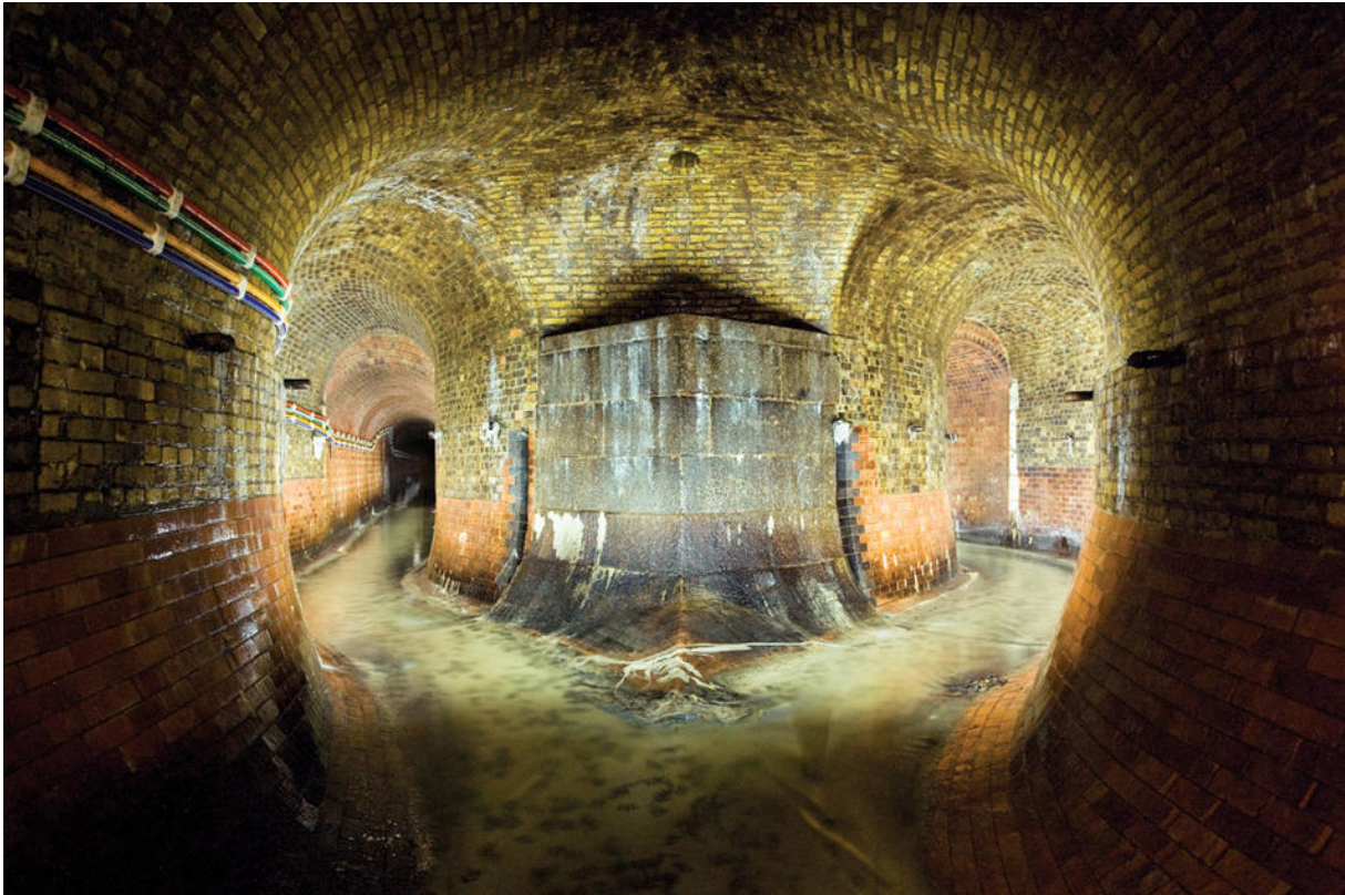
Fleet River sewer, London (Steve Duncan).
