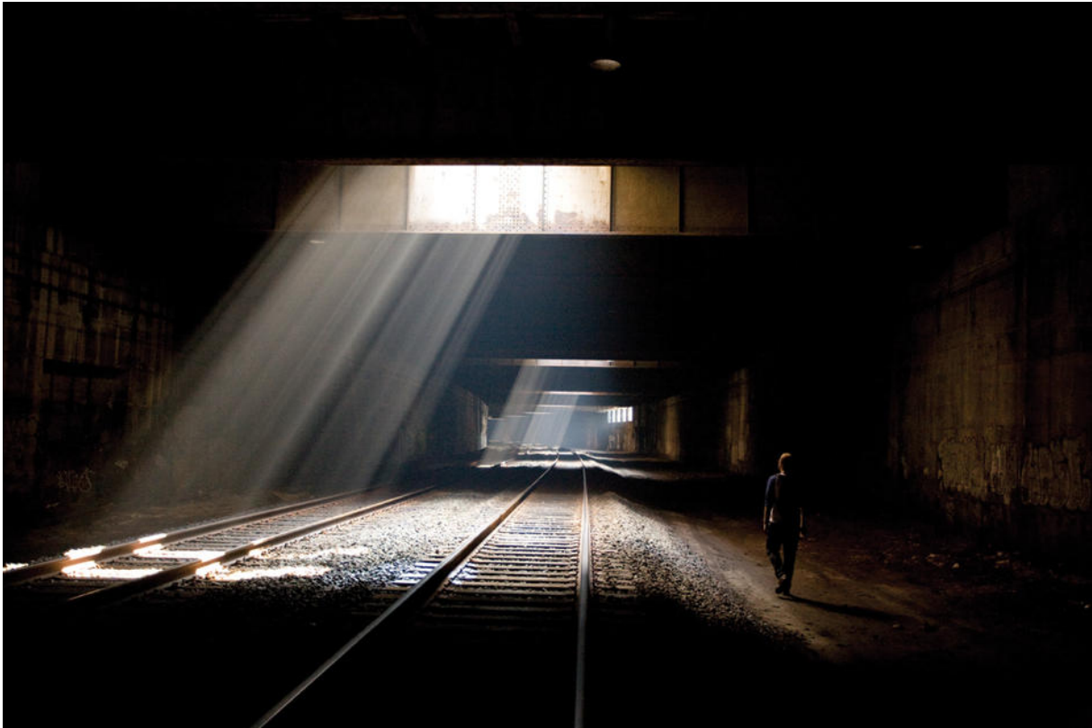
Riverside Park Tunnel, Manhattan (Steve Duncan).
