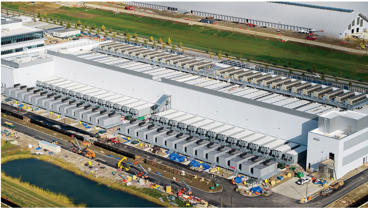
A new data center under construction in Columbus, Ohio. (Snehit Photo / Shutterstock)
