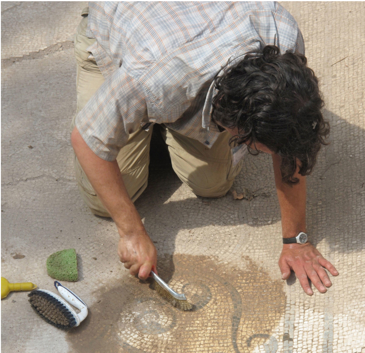
Removing limestone buildup from the surface of the building's mosaic floor. Photo by Francesco De Angelis.
