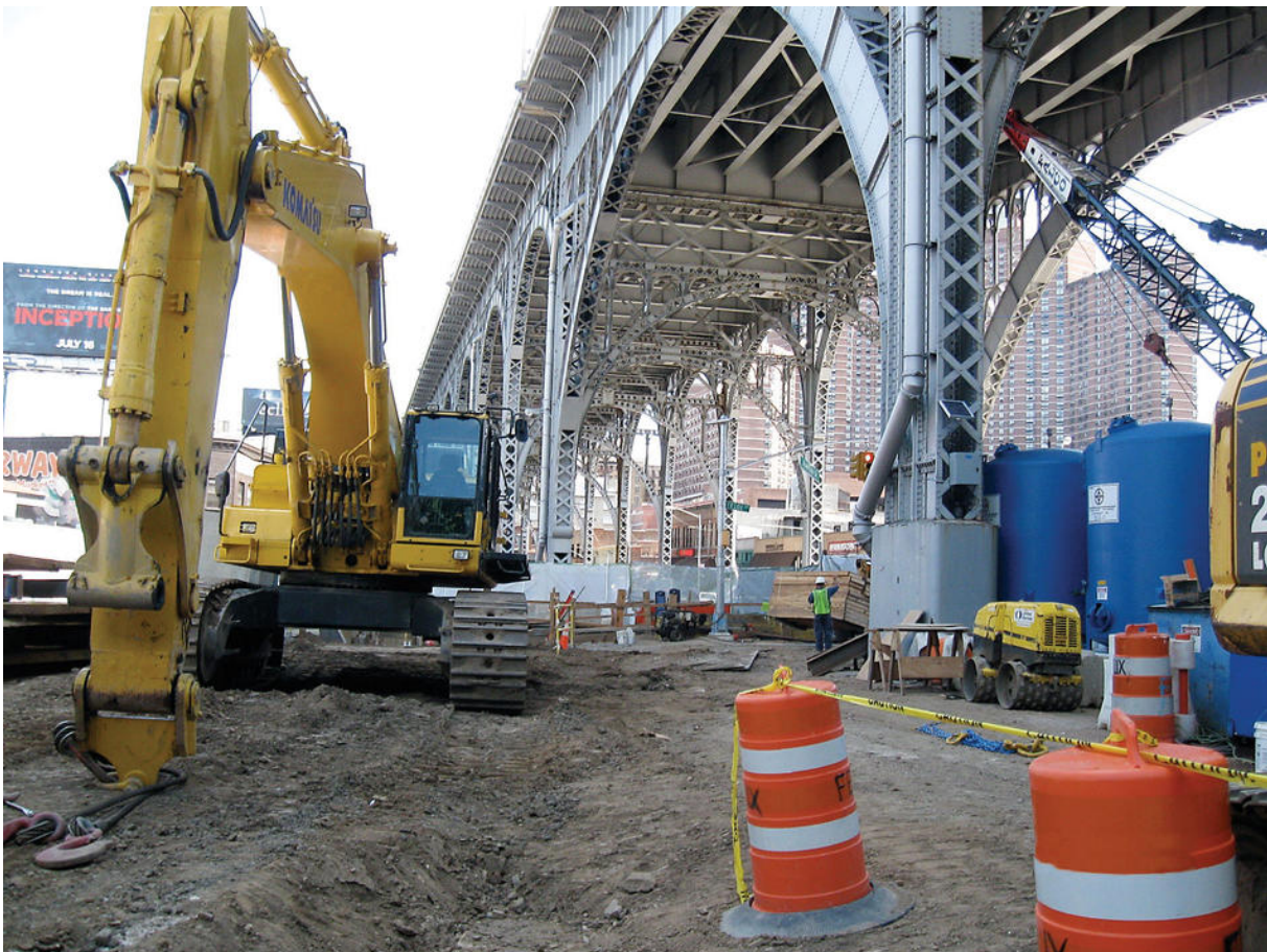
Columbia construction on 12th Avenue, beneath the Riverside Drive Viaduct. (Columbia Facilities)
