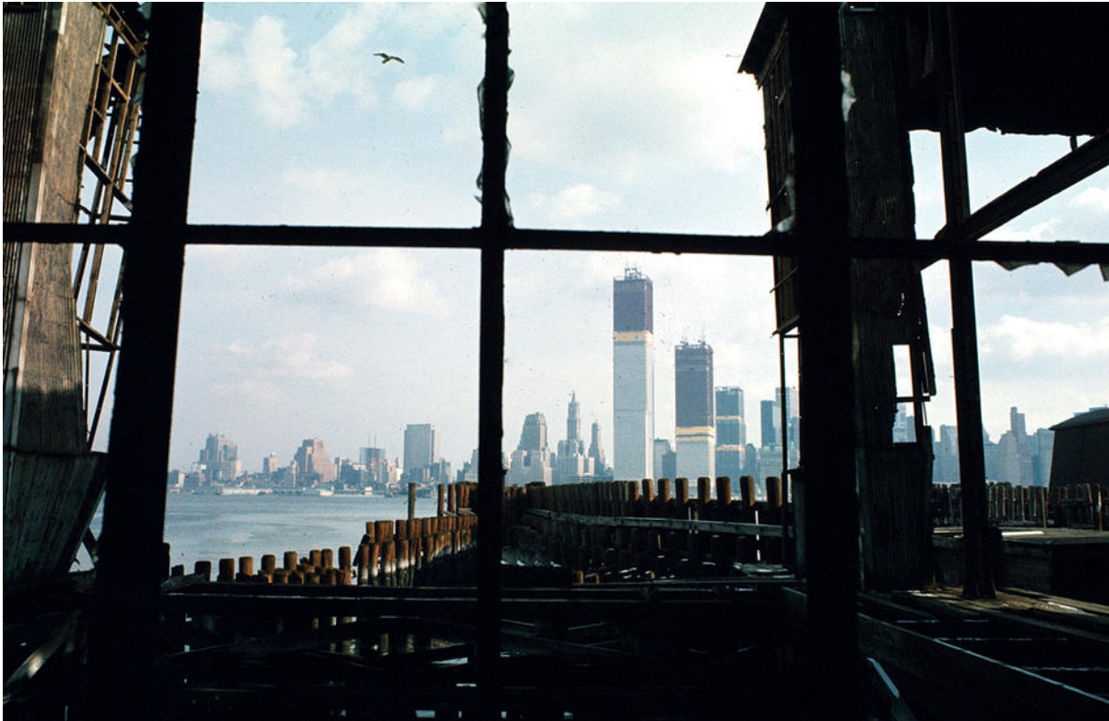
An abandoned pier, Jersey City, New Jersey, 1970. (Camilo José Vergara)
