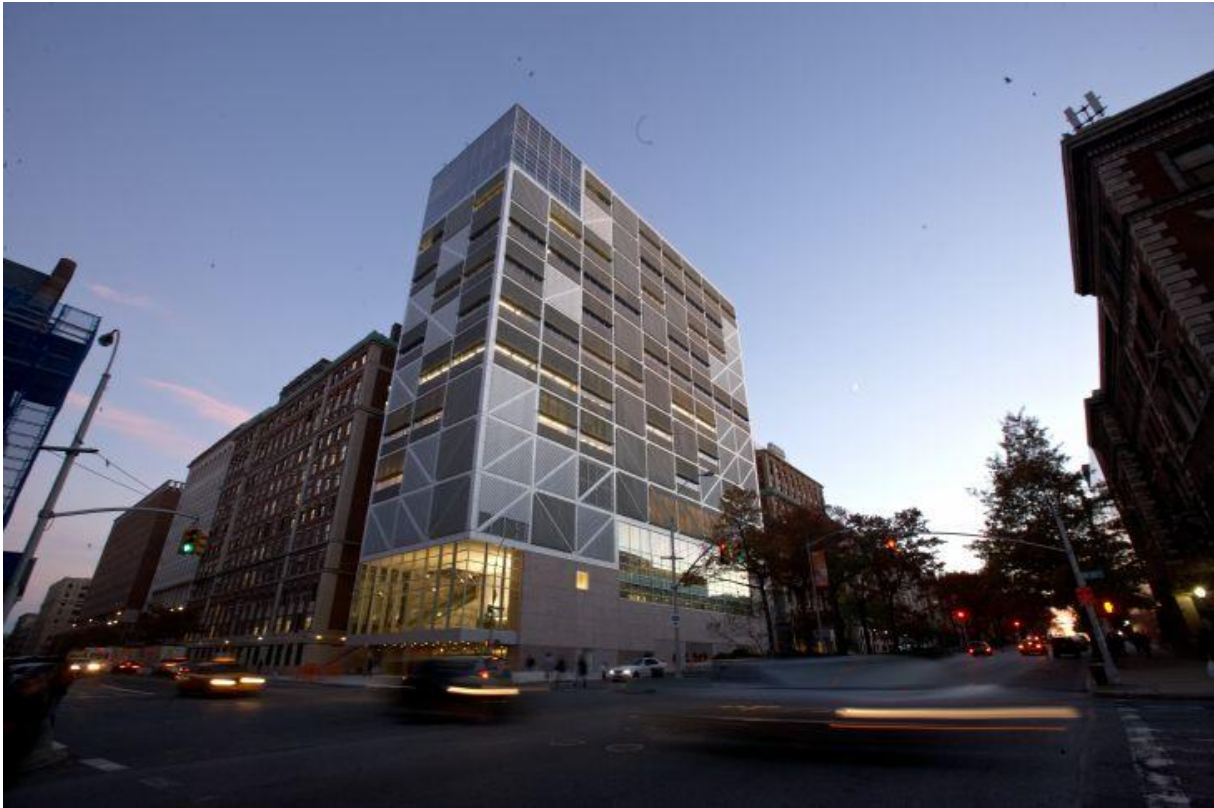
Northwest Corner Building (Bob Handelman, 2010)
