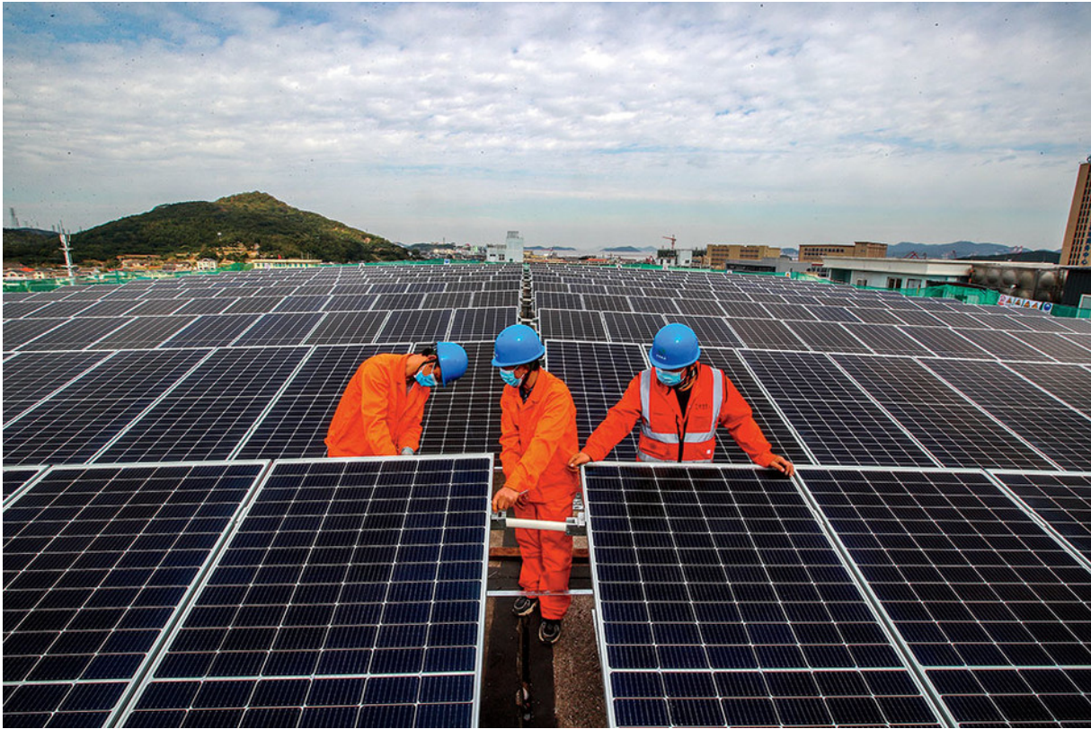
Workers install solar panels on the roof of a fish-processing plant in Zhoushan, China. (Yao Feng / VCG via Getty Images)
