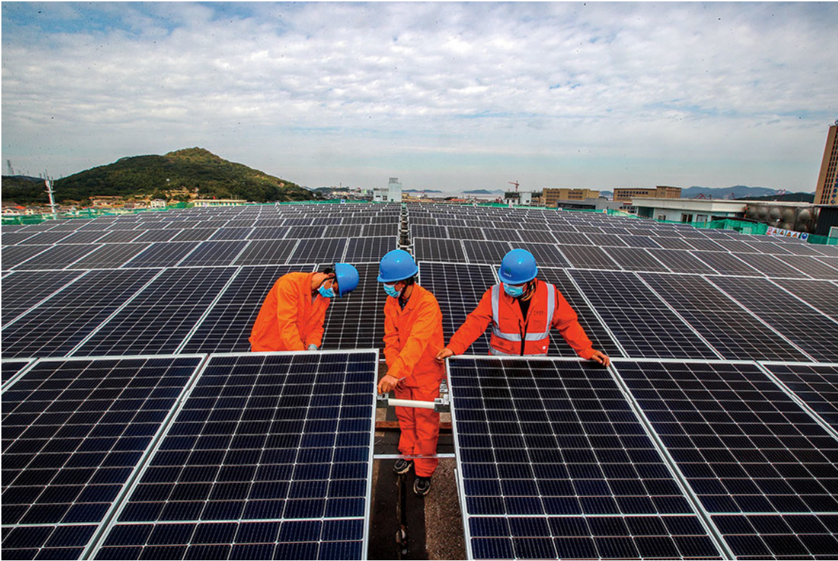
Workers install solar panels on the roof of a fish-processing plant in Zhoushan, China. (Yao Feng / VCG via Getty Images)
