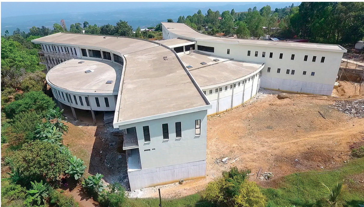
The Women’s Health Pavilion under construction in Kigutu, Burundi. (Manuela Gikoro)
