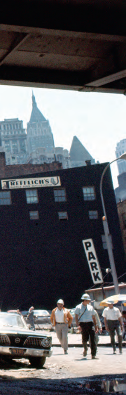
World Trade Center under construction, seen from West Street, Manhattan, 1970
