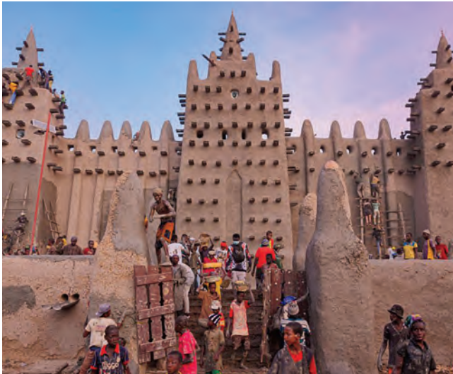
Left: Replastering the Great Mosque of Djenné, in Mali. Right: Rammed-earth buildings in Sana'a, Yemen.
