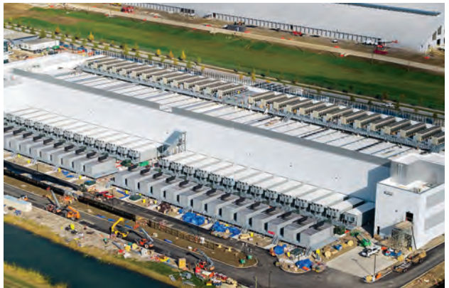
A new data center under construction in Columbus, Ohio.
